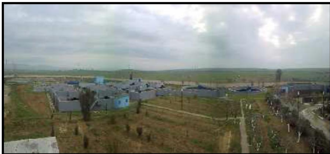
Figure n°5 : La station d'épuration de SBA (ONA, SBA, 2017).
