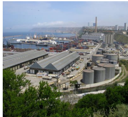
Fig 10. Installation COGO (huile). (EPO,2018).
