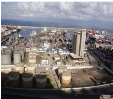
Fig 9. Installation NAFTAL. (EPO,2018).
