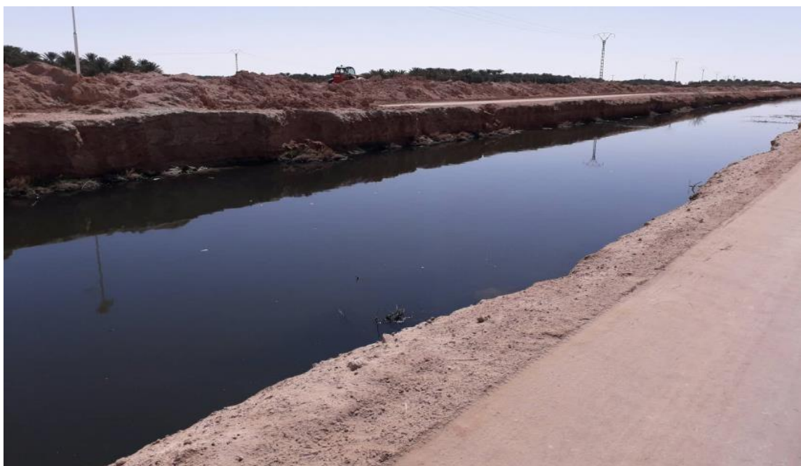
Figure 5 : Canal Oued Righ (Station Touggourt).
