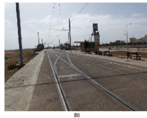
Figure 1. (a) Plan view of the marshy areas (provided by Algiers Metro Company) and (b) photograph of the studied project after the execution phase
