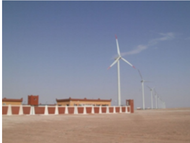
fig. 4.1 – Wind Farm of Kabertene
