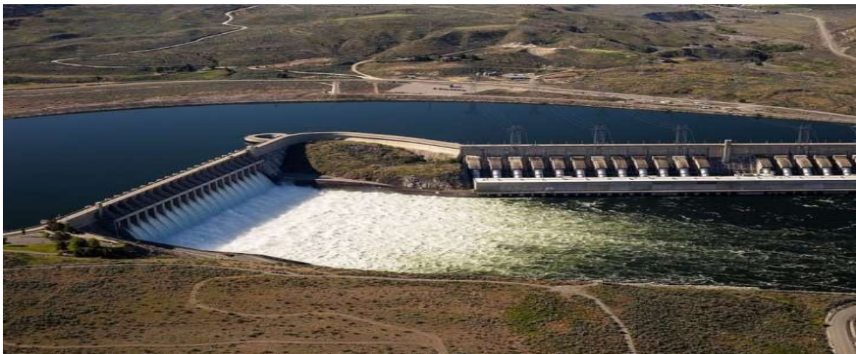
Figure I-2 barrage de Chief Joseph –Washington USA.
